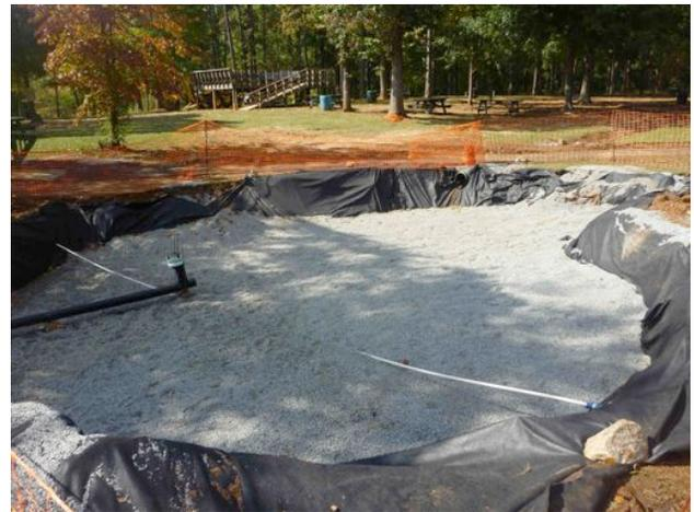
Installation of filter fabric and stone base layer in rain garden.
